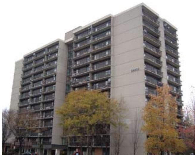
The McDonnell Towers in Southfield were built using MSHDA incentives. MSHDA finances low-income housing across the state, but could be operated more efficiently if leased to a private lender.
