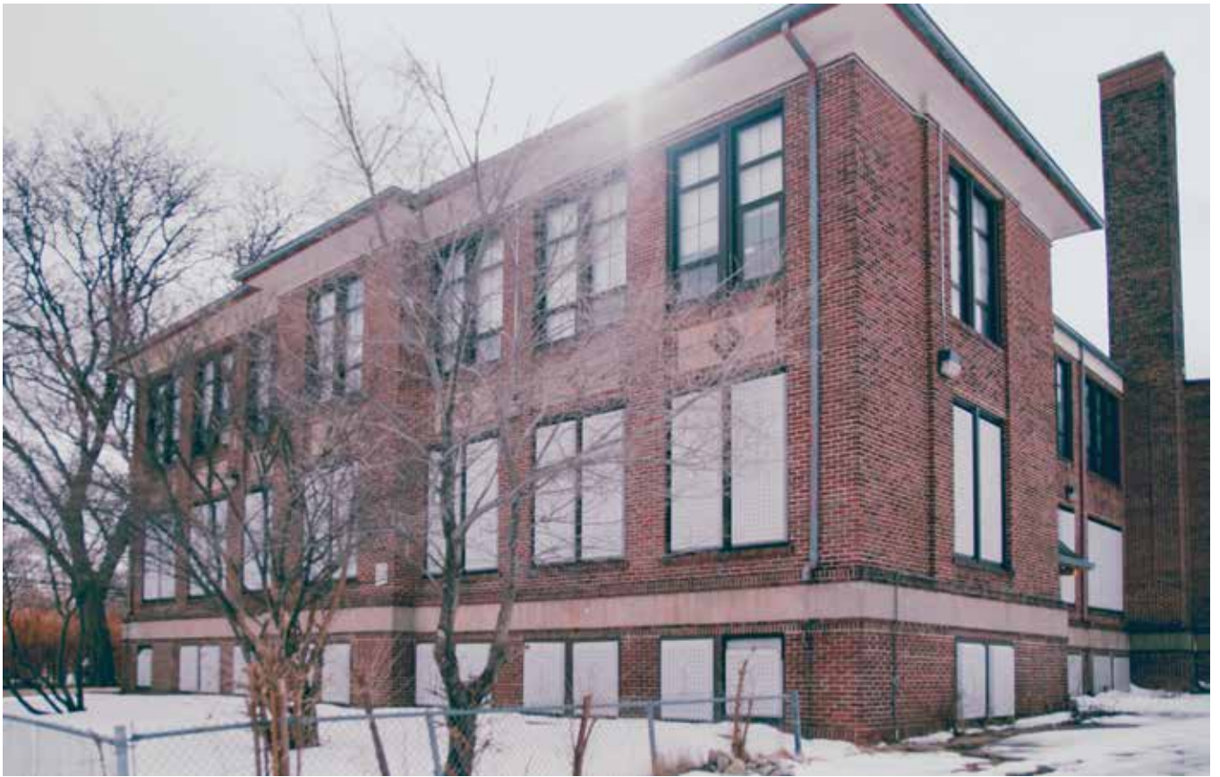
Detroit Prep's new building could support them for years down the road.
