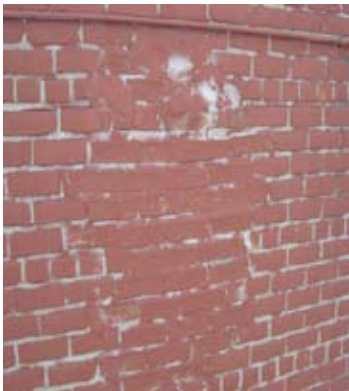
Graphic 19: The Repaired Warehouse Wall of Martin & Snyder Product Sales in Detroit
