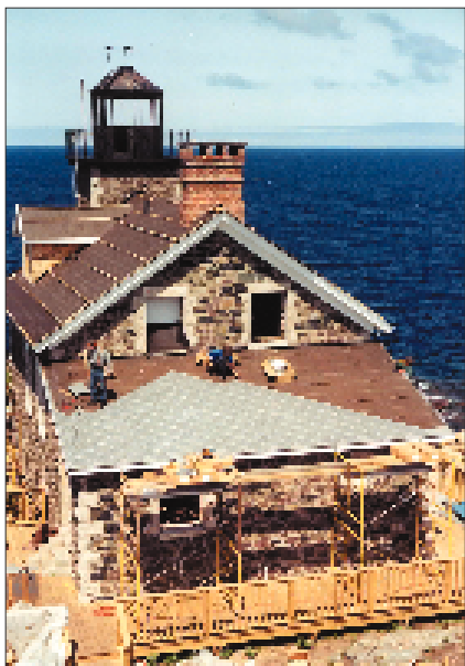
New roofing tiles made of zinc being added to the lighthouse.
